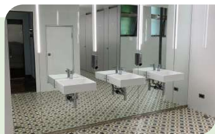
All gender restroom on the first floor of the College of Engineering Building.
