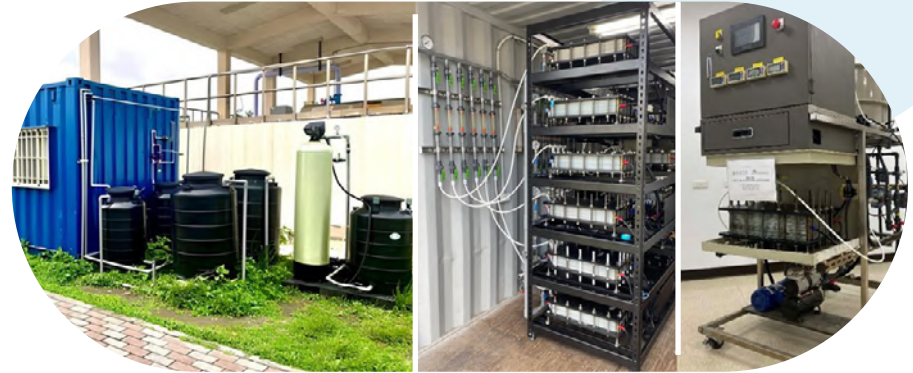
Reclamation at the Keya Water Resources Recycling Center (left and center), and for fluoride-containing semiconductor wastewater treatment and resource recovery (right).
